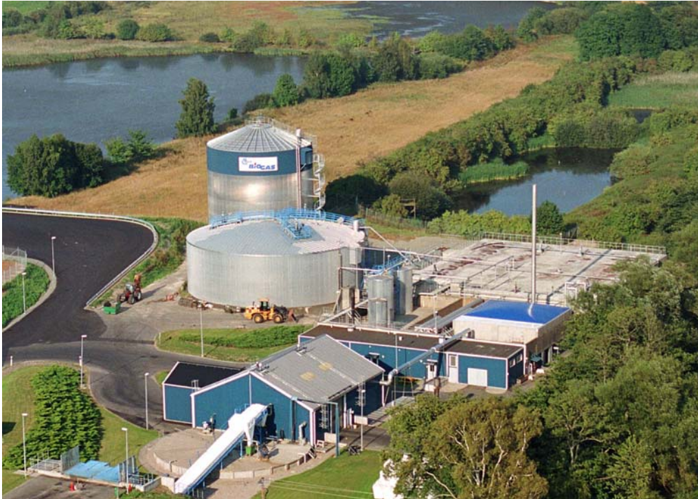
Figure 4.3.1 The biogas plant at Karpalund, Kristianstad
