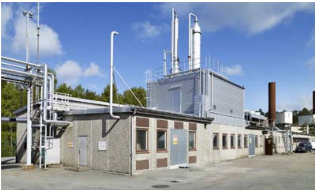
Figure 4.6.1 The upgrading plant at Arendal, Gothenburg
