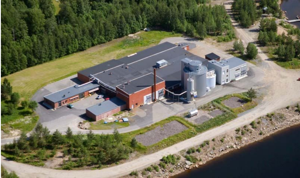
Figure 4.1.1 The biogas plant at Svedjan, Boden
