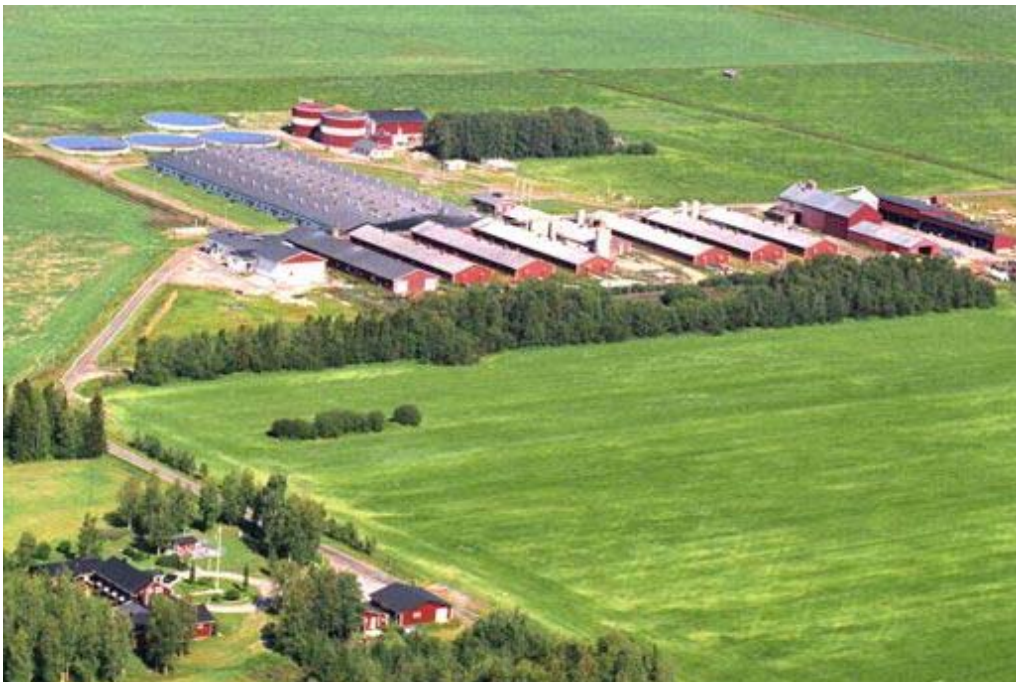
Figure 4.8.1 Photograph of the biogas plant in Alvik
